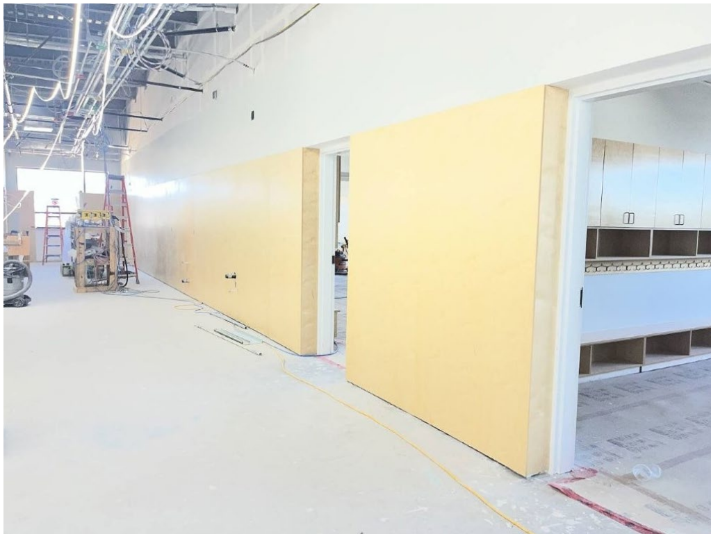
New Addition Millwork Panelling
