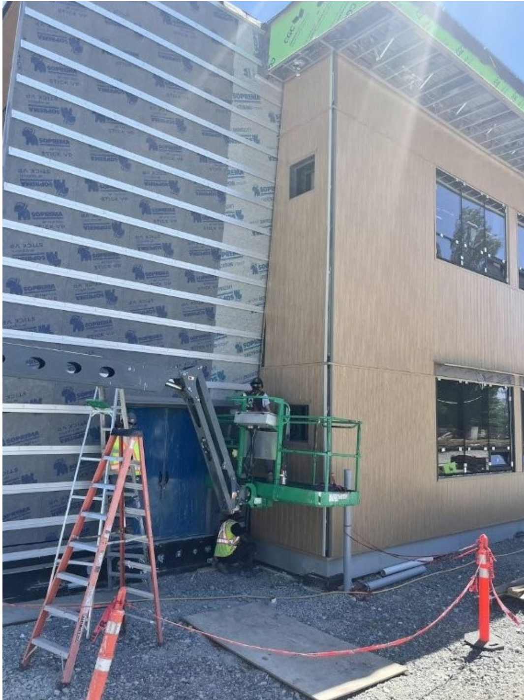
New Addition Angled Wall Cladding
