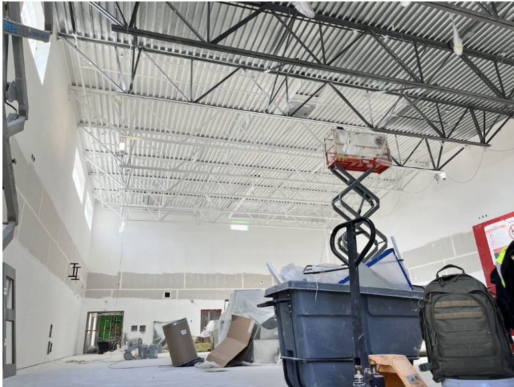
Gym Ceiling Spray Progressions
