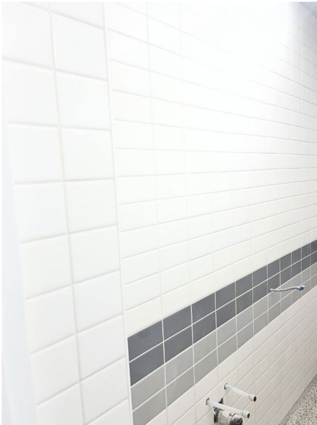
New Addition Washroom Tile Grouting
