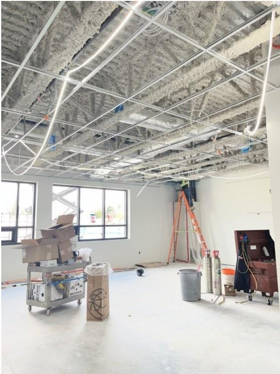
North Addition – Ceiling Tile Grid
