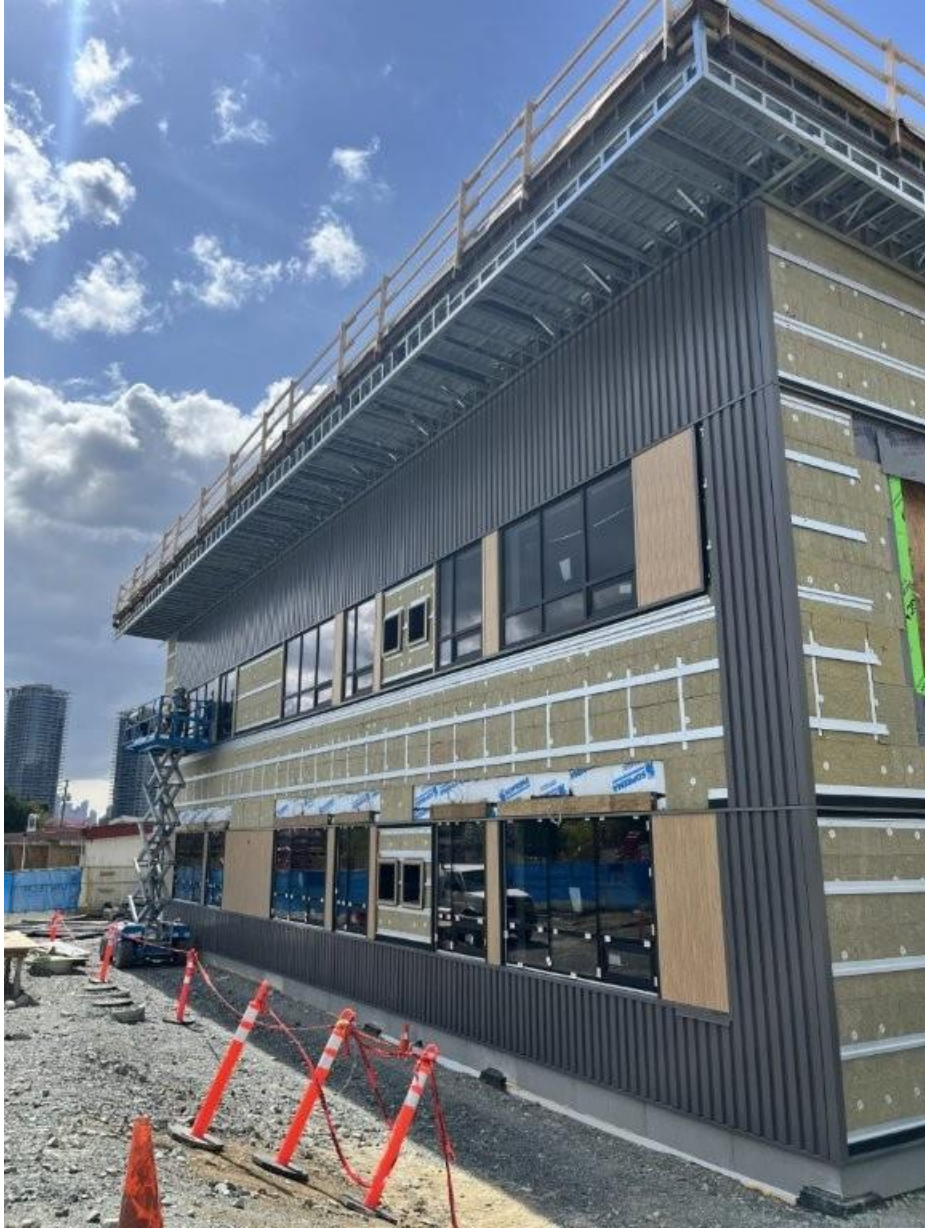
North Addition – Cladding Panels
