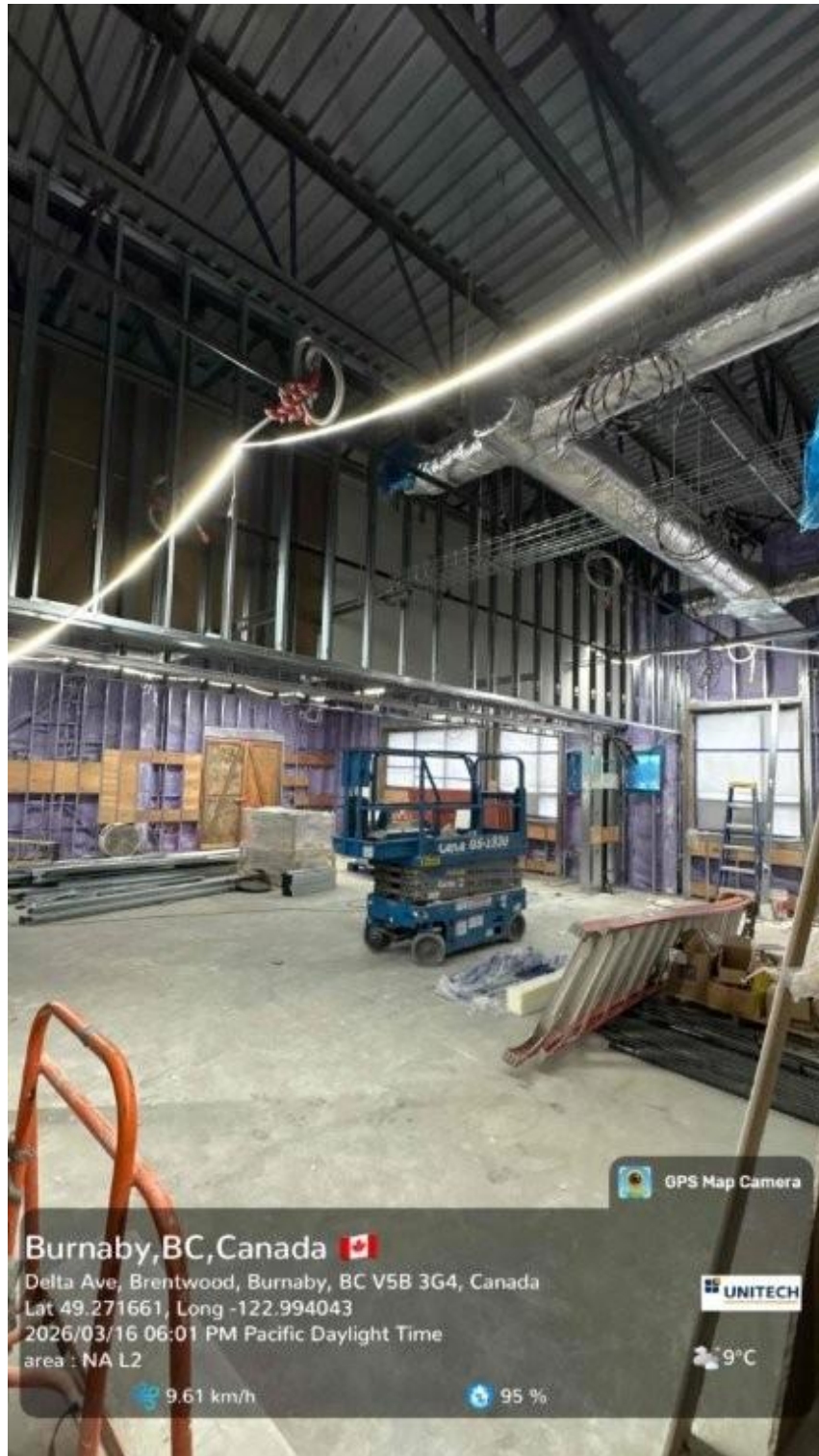
North Addition – Level 2 Classroom Interior
