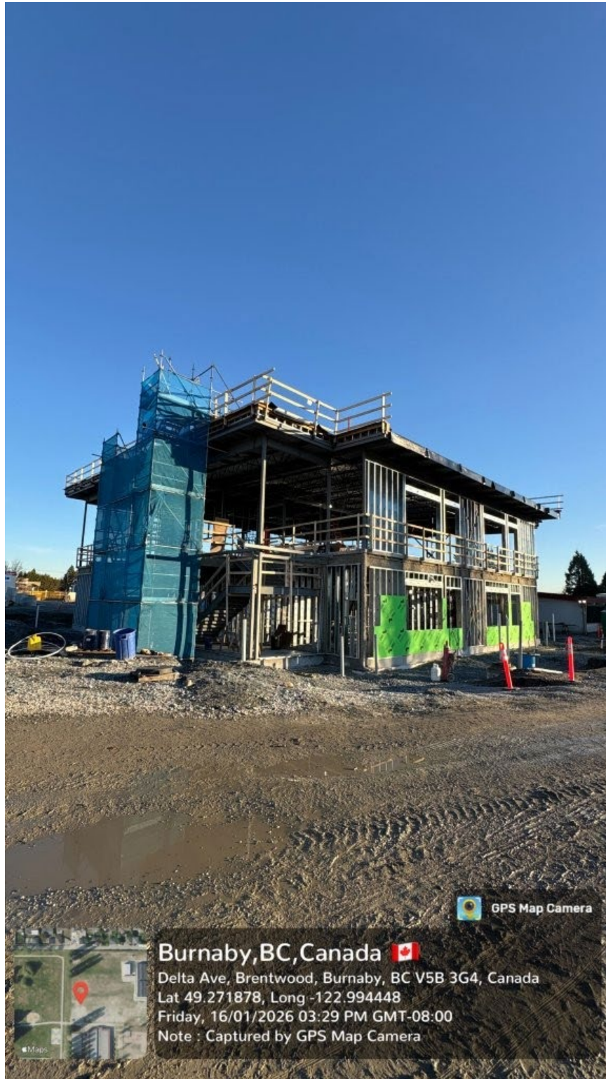
New Classroom Addition – Steel Stud Framing
